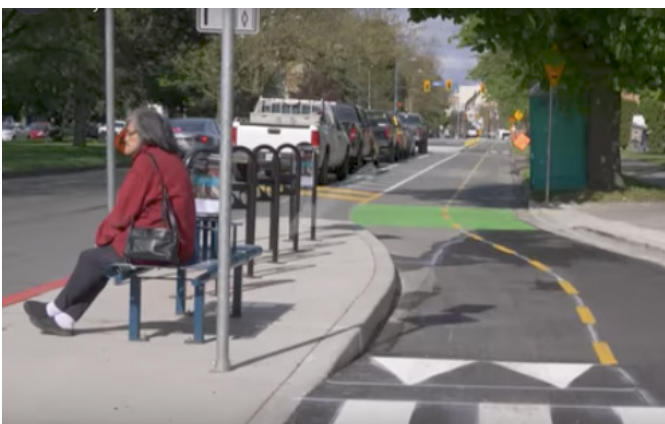
Figure 5: Floating Bus Stop on Pandora Avenue. Credit: City of Victoria
