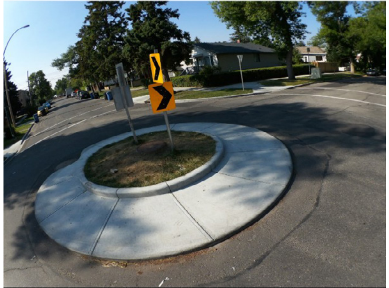
Figure 28: Roundabout traffic island on 8th Avenue NE, Calgary, AB; Credit: City of Calgary
