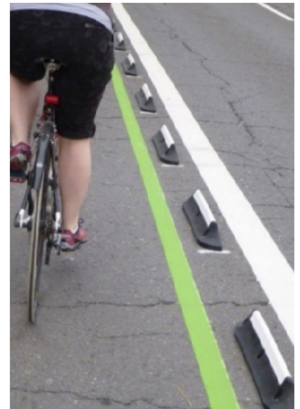
Figure 10: Rubber curb separation along Cannon Street cycle tracks, Hamilton, ON. Credit: City of Hamilton
