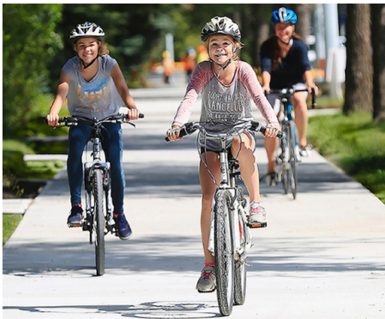
Figure 29: Concrete shared-use path on 102nd Avenue, Edmonton, AB; Credit: City of Edmonton
