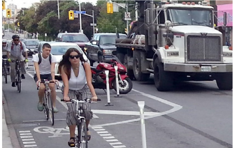
Figure 1: Bollard protected cycle track on Bloor Street, Toronto, ON. Credit: City of Toronto
