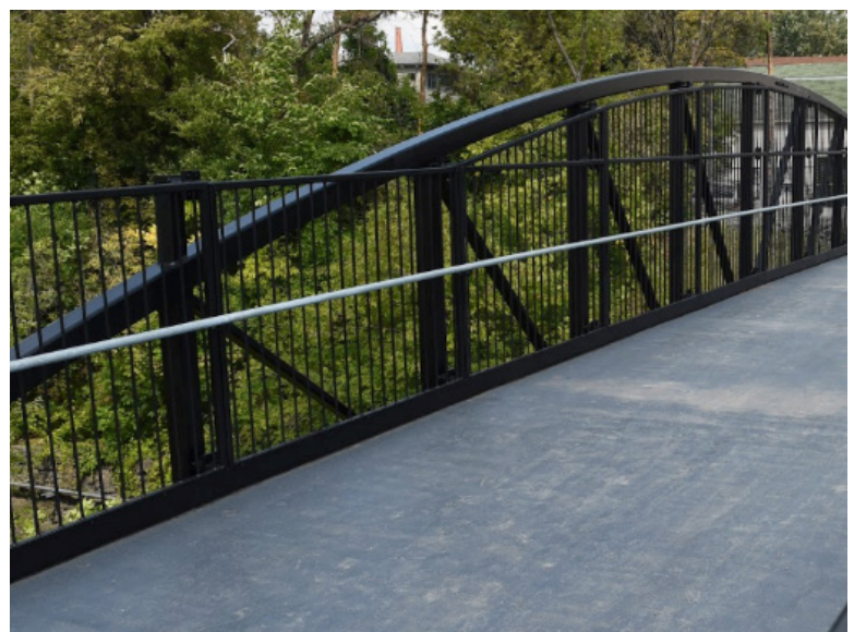
Figure 31: Hickory Street Bridge, Ottawa, ON; Credit: City of Ottawa
