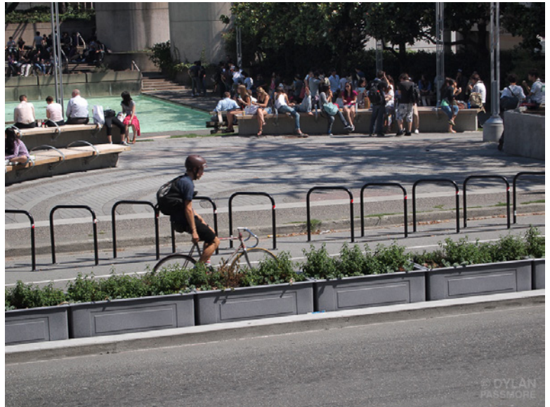
Figure 7: Concrete median protected cycle track with planting on Dunsmuir Street, Vancouver, BC. Credit: Dylan Passmore
