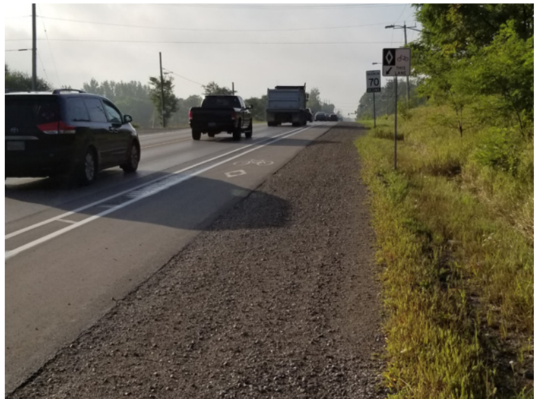
Figure 11: Victoria Road with buffered rumble strips, Guelph, ON. Credit: City of Guelph
