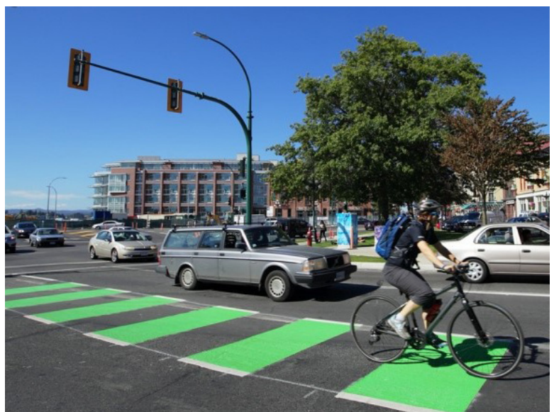
Figure 12: Dedicated painted bicycle lane on Johnson Street, Victoria, BC. Credit: Times Colonist
