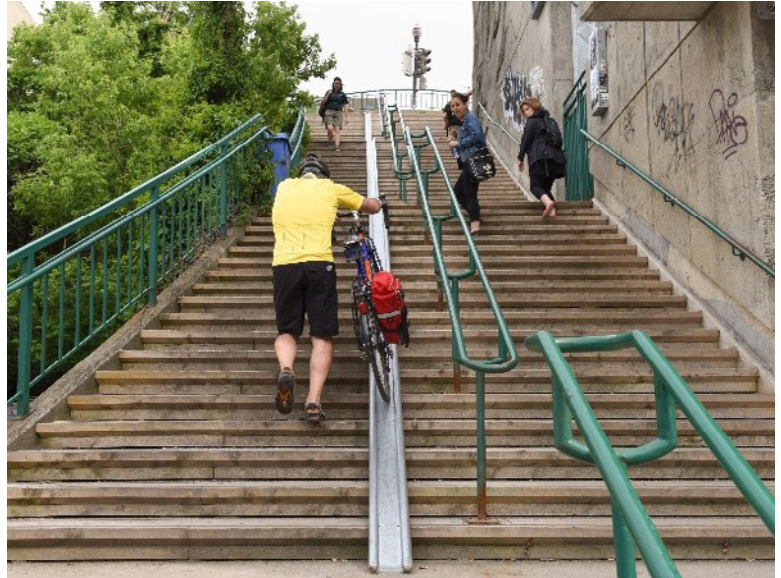
Figure 42: Stairway Channel, Quebec City, QC; Credit: Ville de Québec
