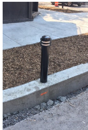
Figure 24: Bollard installed on a Montreal curb extension; Credit: Julia Malmo-Laycock
