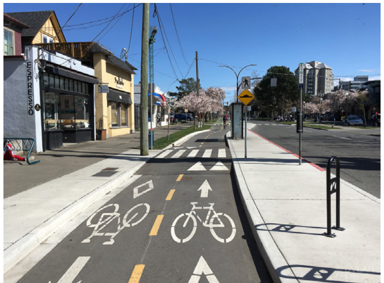
Figure 3: Concrete median protected cycle track on Pandora Ave in Victoria, BC. Credit: Dylan Passmore
