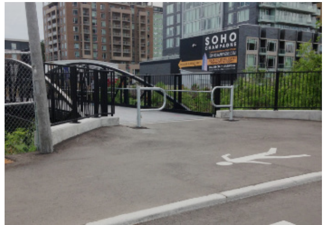
Figure 32: Hickory Street Bridge abutments, Ottawa, ON; Credit: City of Ottawa
