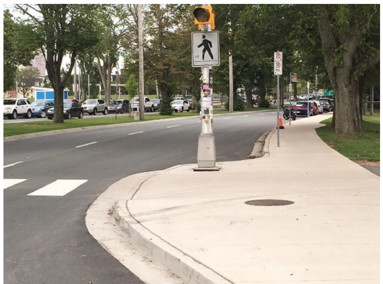
Figure 21: Concrete curb extension on Cogswell Street, Halifax, NS; Credit: City of Halifax
