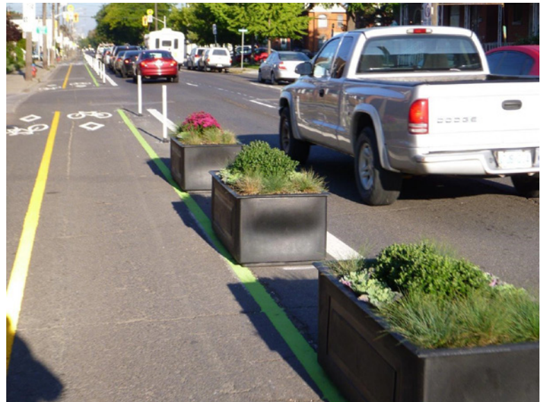
Figure 9: Protected cycle tracks with modular planters on Cannon Street Pilot, Hamilton, ON. Credit: Norma Moores, IBI Group
