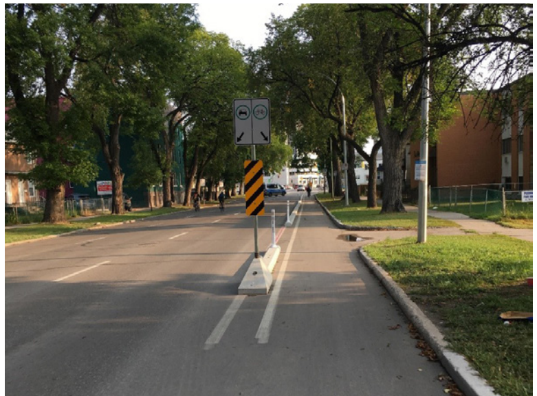
Figure 2: Adjustable concrete barrier protected cycle track on Sherbrook St, Winnipeg, ON. Credit: City of Winnipeg
