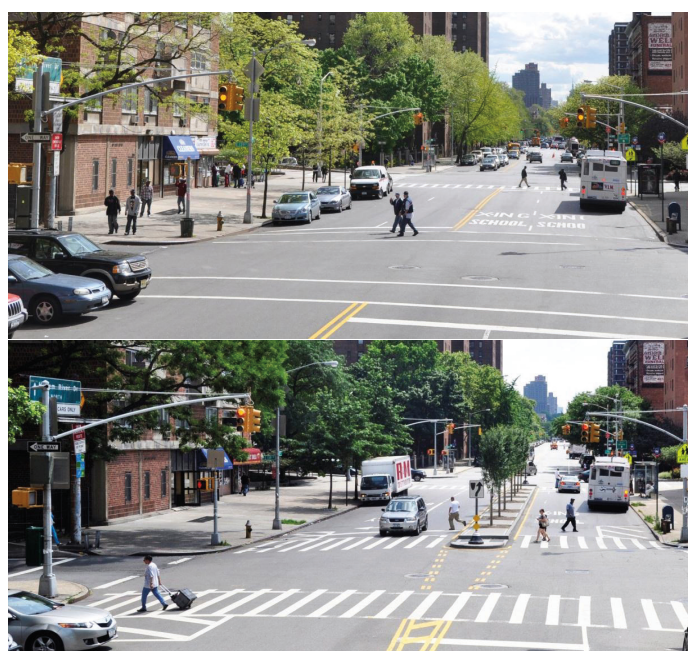
Before and after photos of 5th Avenue in New York City, following the installation of clear paint markings and a centre median. Source: Sean Quinn.
