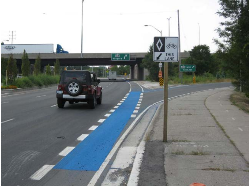
Figure 5- Completed Fairview Interchange
